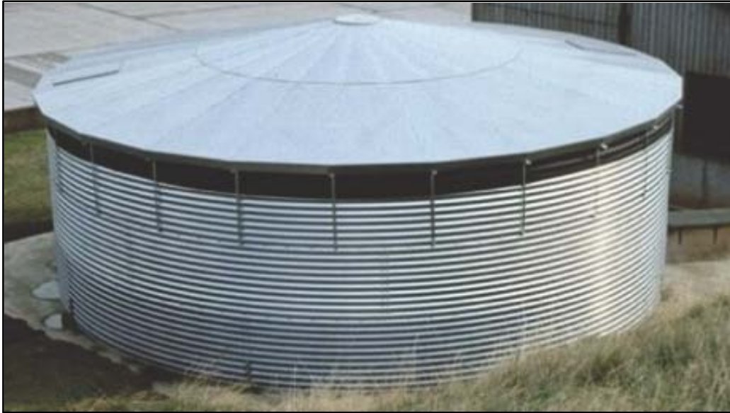
Photograph 1 – 450,000 litre water tank
